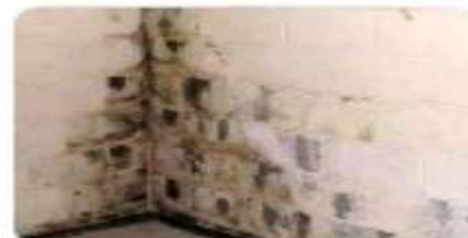
WHITE MOLDS IN BASEMENT
