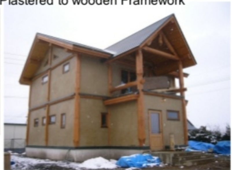
Mud being Plastered to wooden Framework
