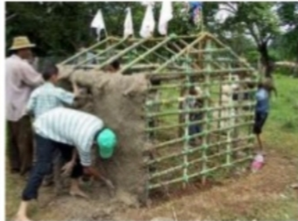
Mud being Plastered to wooden Framework
