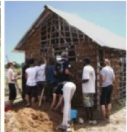
Mud being Plastered to wooden Framework
